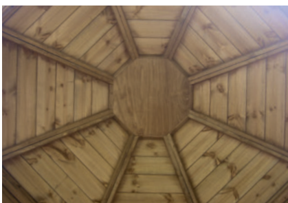
Internal roof structure
