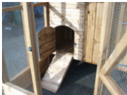
Hen access door and ramp
