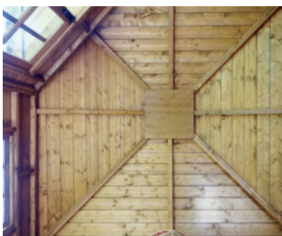
Internal roof structure
